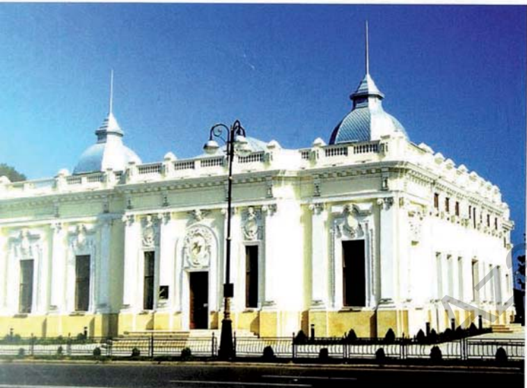
The Abdulla Shaiq Azerbaijan State Puppet Theatre (former Phenomenon Cinema). 1912, design by J. K. Plushko. Substantial reconstruction and renovation was undertaken in 2007.
